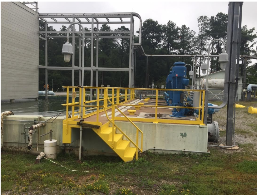
Figure A.4 System Pumping Platform
